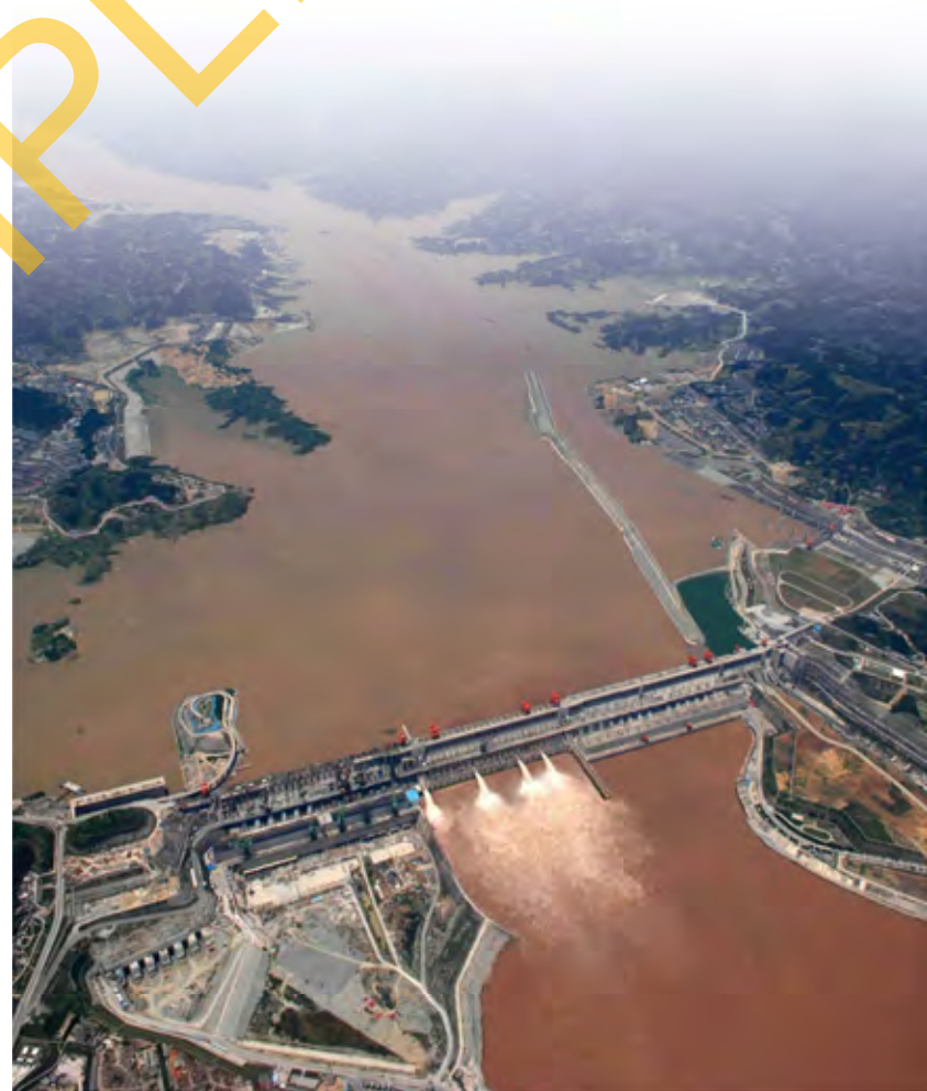
Source 1.26 An oblique aerial view of the Three Gorges Dam on the Yangtze River in China. Water flows through the open sluice gates. The hydroelectric power station is to the left of the sluice gates.
