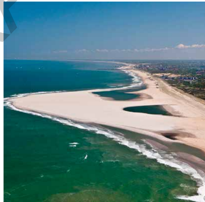
Source 2 In the Netherlands a vast sand peninsula 2 kilometres long and 1 kilometre wide has been constructed. Dubbed the 'sand engine', waves and currents are redistributing the peninsula along the shore where it is expected to nourish the beaches and form sand dunes.
